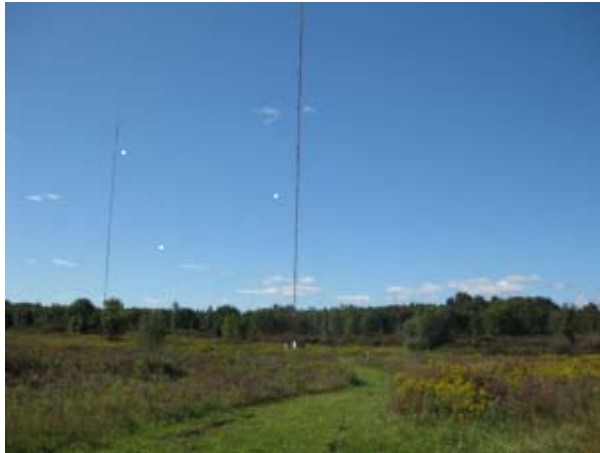
Typical transmitter site
